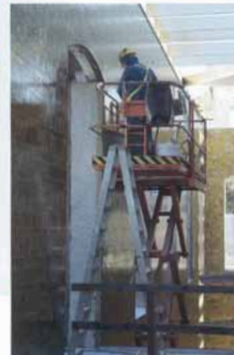
Completamento interno delle murature originarie mediante installazione del rivestimento interno in elementi vetri retroilluminati Completion of the internal masonry with the installation of an internal finish made of glazed back-lit elements
