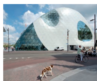
23. Admirant Entrance Building
